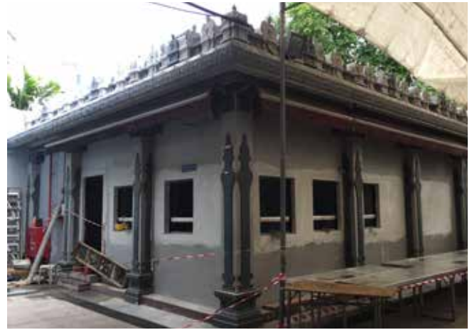
Works on-going for the Temple office to make it more user-friendly
